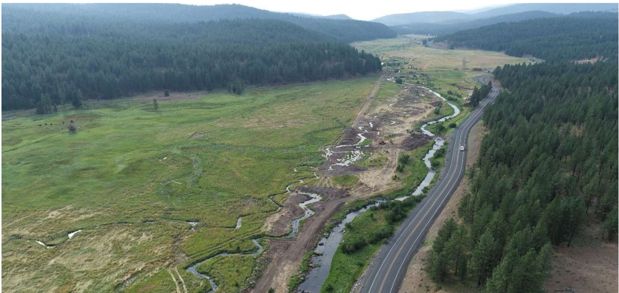
▲ Photo 5. Middle Fork John Day River restoration work completed by the Confederated Tribes of Warm Springs.
